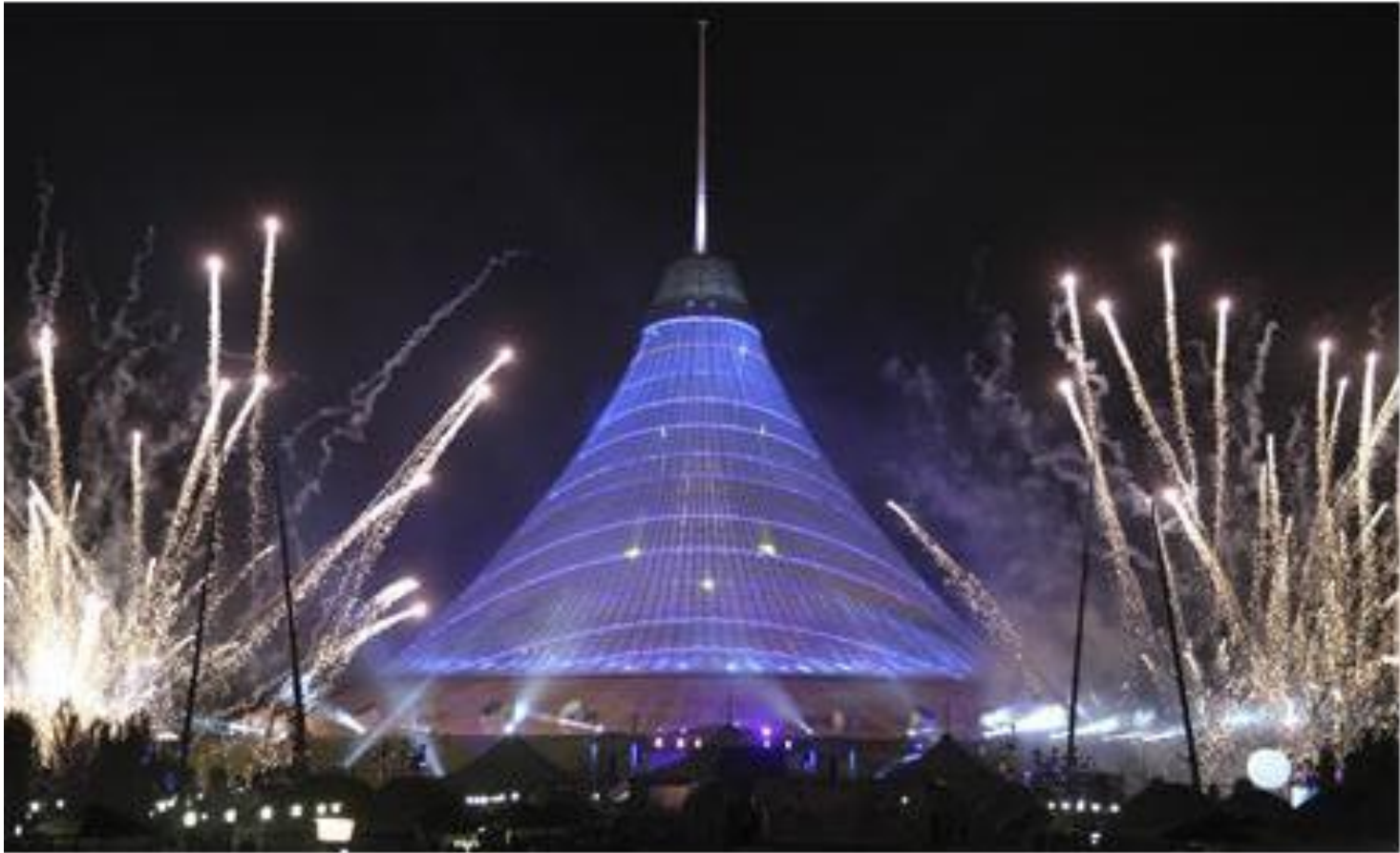
Khan Shatyr, billed as the world's biggest tent and built by Turkish hotelier and construction magnate Fethi Tamince and his partners, is seen after its opening in Astana July 6, 2010.
