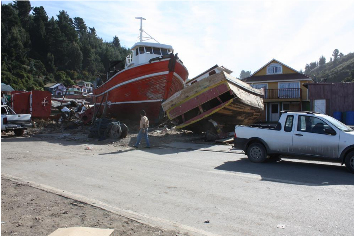
Tsunami damage at Caleta Tumbes, north of Concepción
