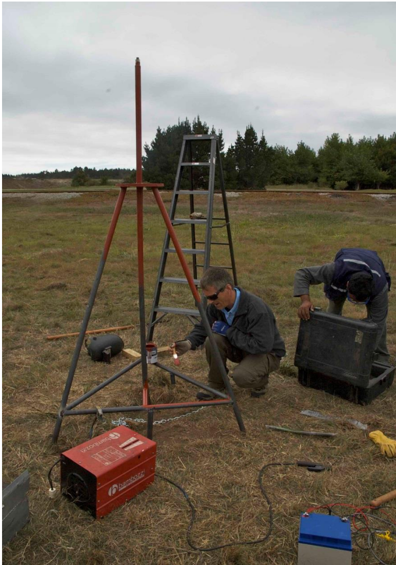
Applying anti-corrosion paint
