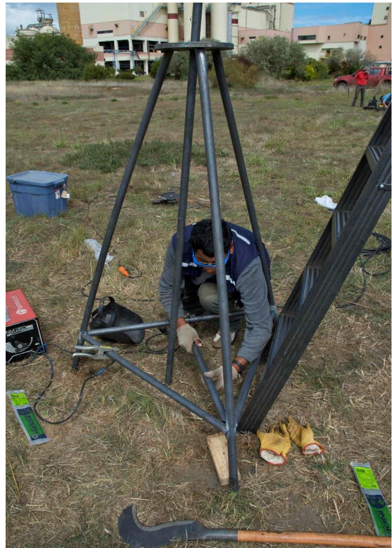
Fitting the support for the upright bar
