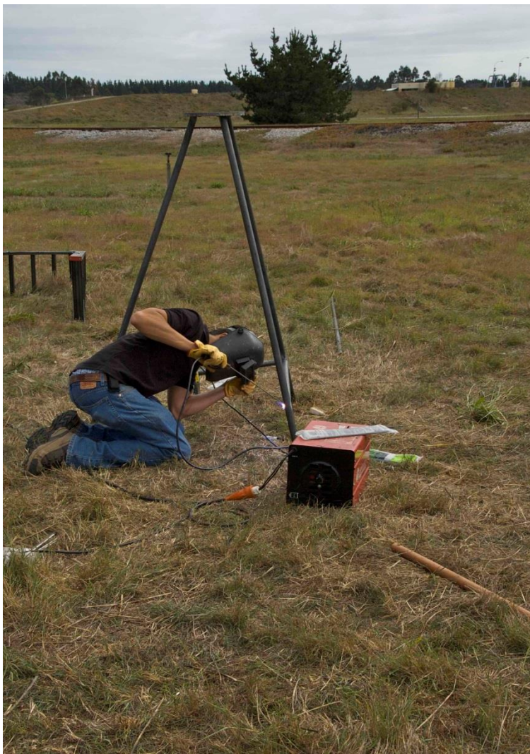
Welding the triangular bracing
